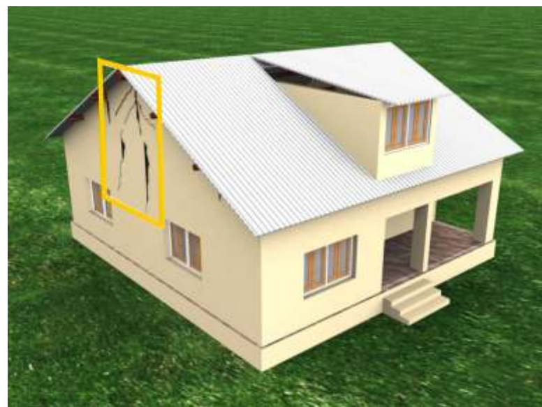
Cracks at floor and ridge beam support
